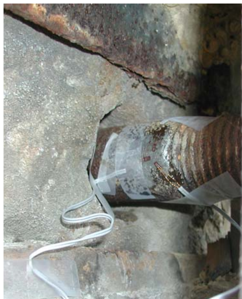
Figure 3: Strain gauges applied to tie-rod
