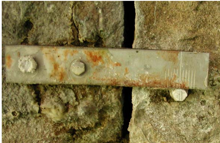
Figure 2: Crack gauge installed on bridge 1
