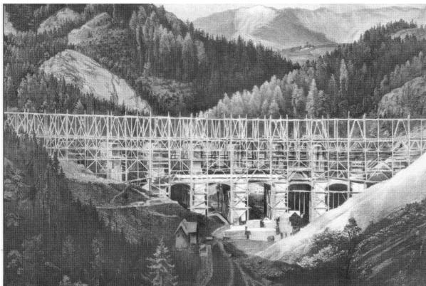
Figure 6: the building of the Kalte Rinne viaduct (Rampati, 2002)
