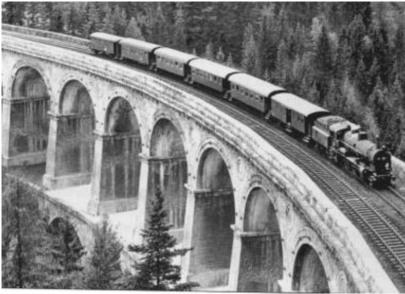
Figure 8: train on the Semmering viaduct (Rampati, 2002)
