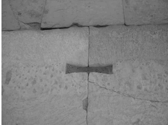
Figure 1 : Joint at Kom Ombo Temple (Egypt)
