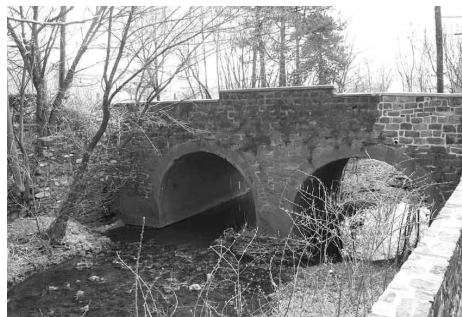
Figure 2: Photograph of Center Street Bridge, Newtown, PA. Constructed 1796, altered in 1875 (PennDOT).
