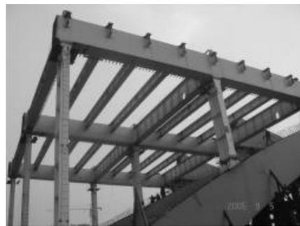
Fig.4: The Latticed Deck Beams
