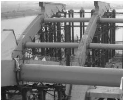
Fig.3: Erection of Side Span Arch Rib
