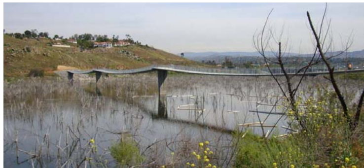
Figure 1 : Lake Hodges Pedestrian Bridge
