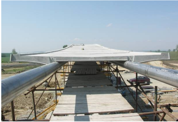
Figure 2 : Segments on external cables
