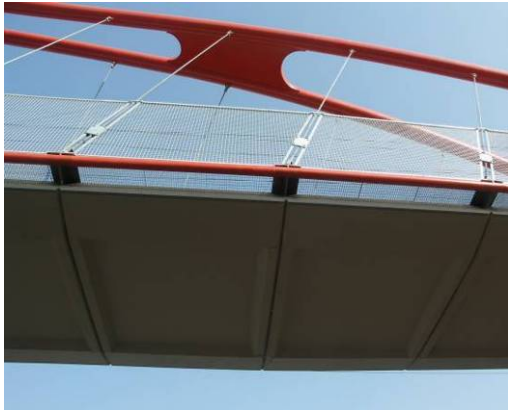
Figure 11 : Suspension of the deck
