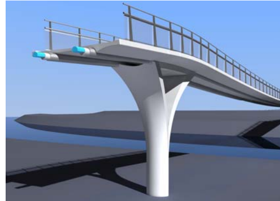
Figure 3 : Stress ribbon & Pier table
