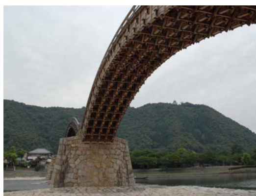
Figure 6 : Wooden framework of Kintaikyo Bridge
