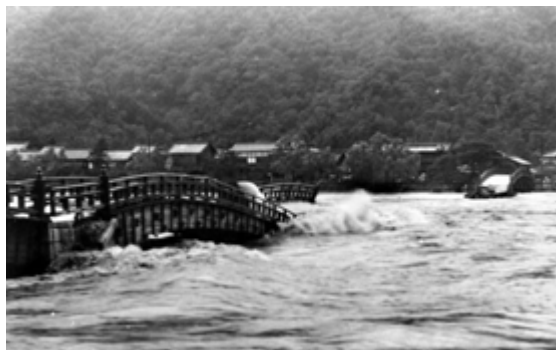
Figure 4 : Arches being washed away
