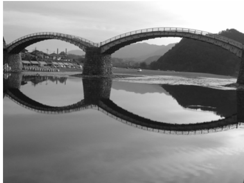
Figure 7 : Form of the arch (Catenary curve)
