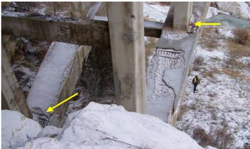
Figure 5 : Cracks and peeling of concrete on arch
