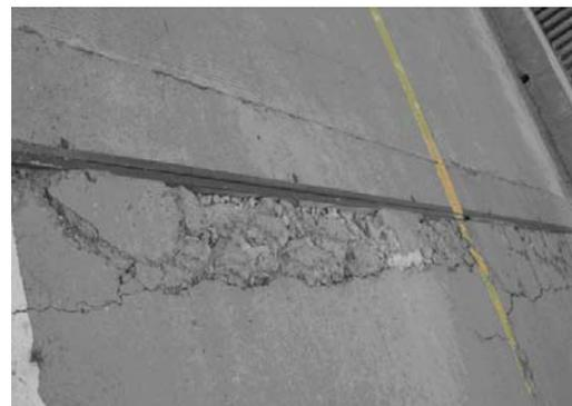
Figure 14 : Deck crush close to expansion joint
