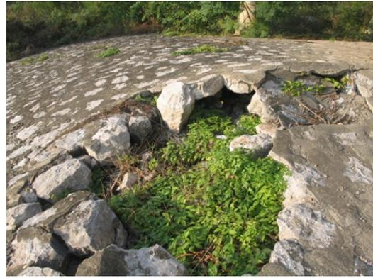
Figure 11: cracks and water seeping on skewback    Figure 12: sink and crush on conical slope
