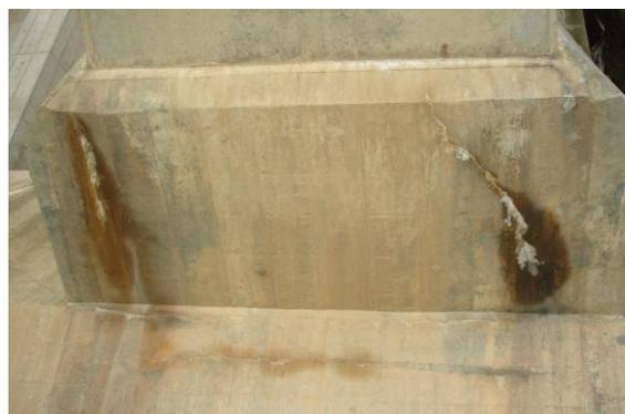
Figure 8 : cracks and water seeping on springing
