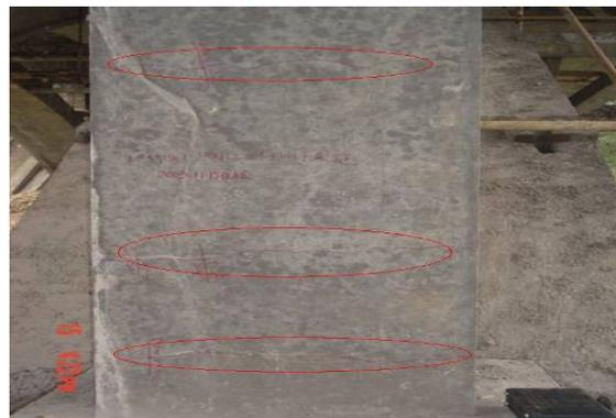
Figure 10 : horizontal cracks on pilars
