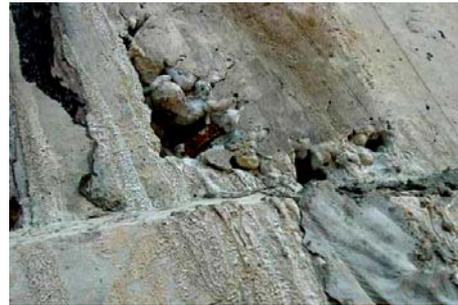
Figure 6 : Broken arch ribs
