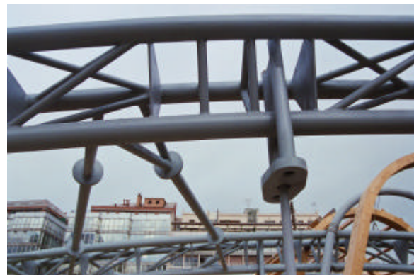
Photo 7 and 8 – Union of hangers to the arches and anchorage of the braces
