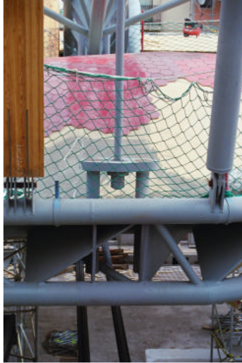
Photo 9 - Union of the hangers to the steel beams
