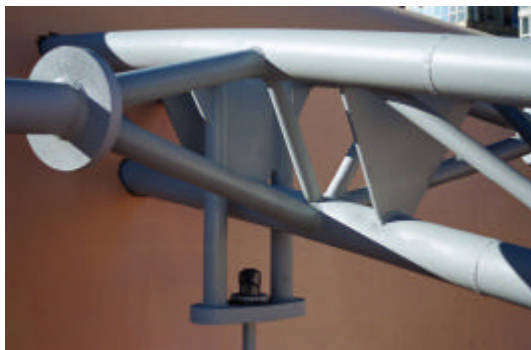
Photo 7 and 8 – Union of hangers to the arches and anchorage of the braces
