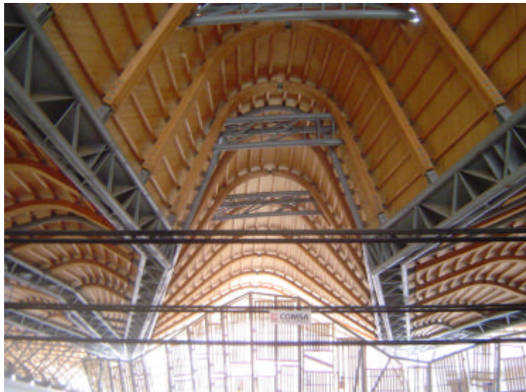
Photo 13 - General view indoors
