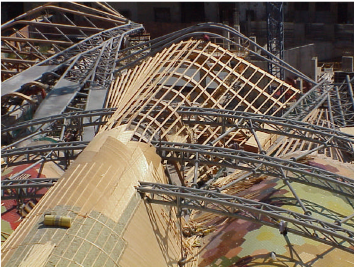
Photo 1 - General perspective under construction
