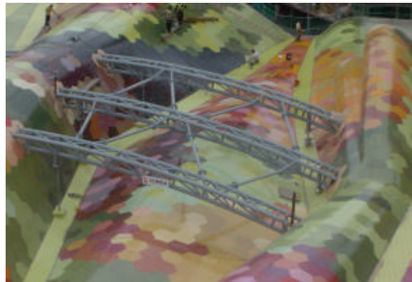
Photo 6 - Bracing of the Arch's
