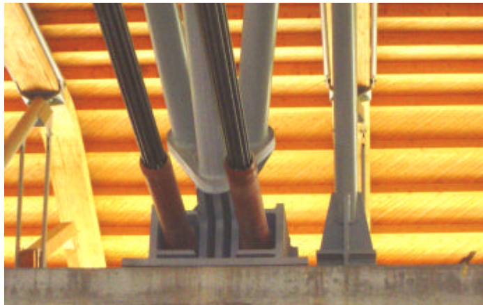
Photo 3 - Supports at the arches
