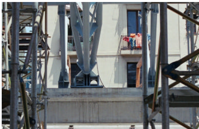
Photo 4 - Supports of the arches
