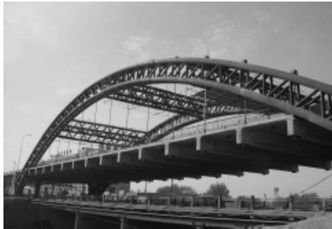
Figure 1: The Beichuan River CFST arch bridge
