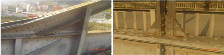
Fig. 4. The capped rivet connections.
