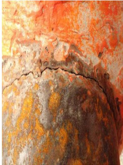
*Fig. 4. Example of crack.*
