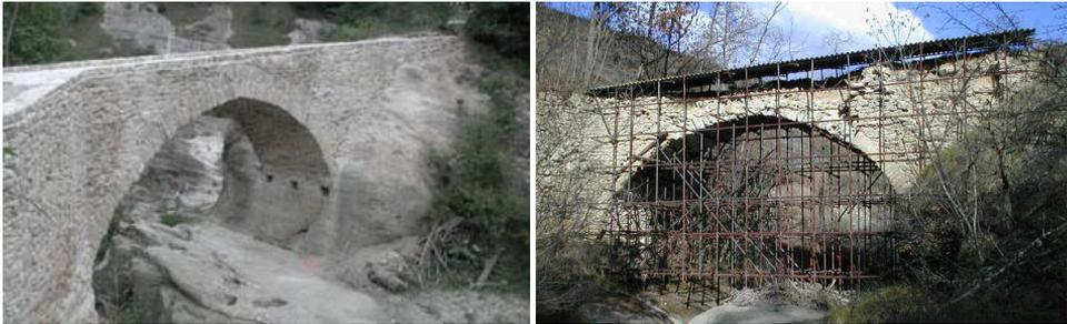
*Fig. 11. The masonry bridge of Sogliano al Rubicone, before and after the consolidation with RAM Method.*
