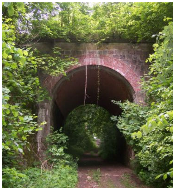
Fig. 4. Viaduct covered by foliage.
