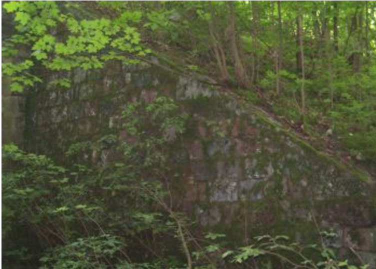
Fig. 9. Stone wing before cleaning and repair.
