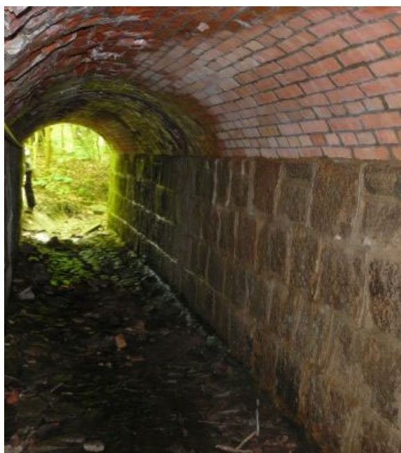
Fig. 5. Masonry culvert.
