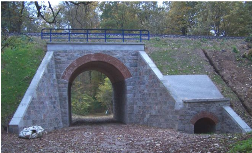
Fig. 6. North elevation of the masonry arch structure after retrofitting
