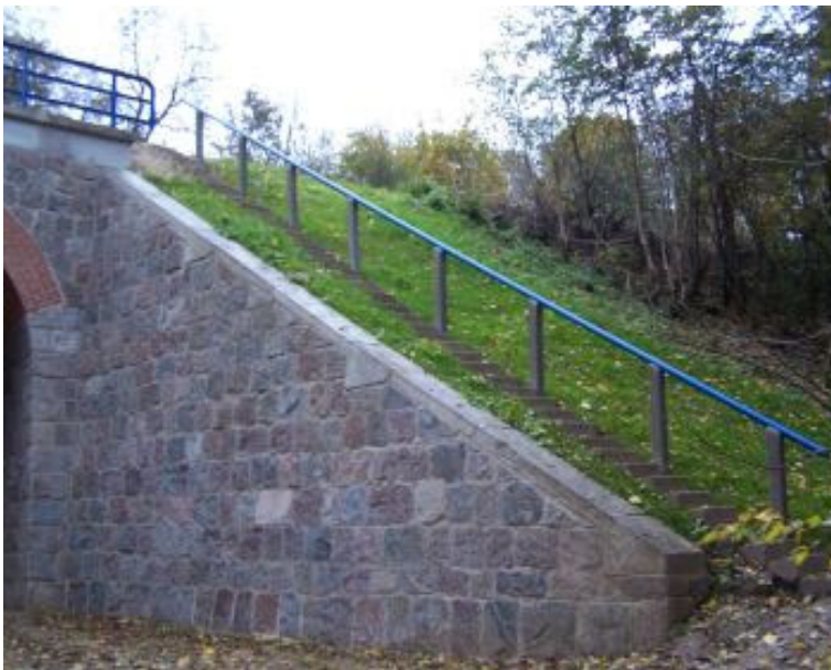
Fig. 10. Stone wing after cleaning and repair.
