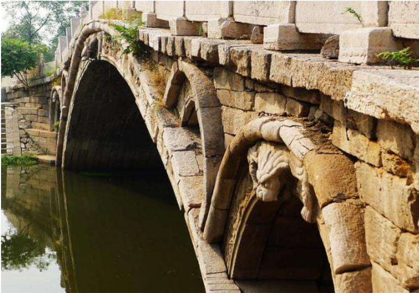
*Fig. 7. The stones seriously weathered and eroded.*
