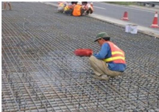
*Fig.12. Replace the bridge deck pavement.*
