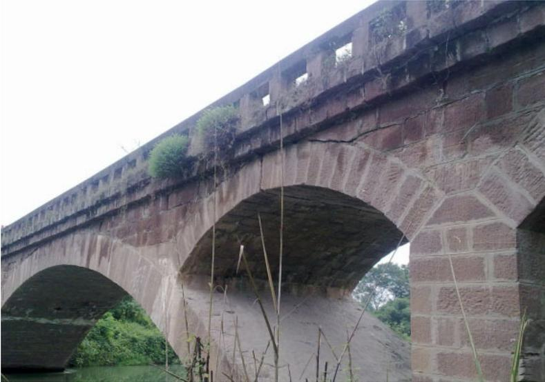
*Fig. 4. The side wall leaning outwards.*
