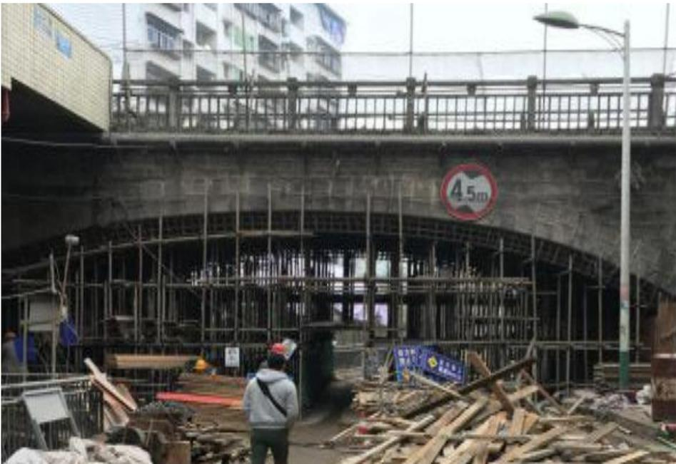
*Fig. 10. Hooped with reinforcement concrete.*
