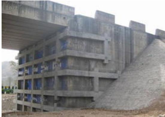
*Fig. 11. Hooped by a frame beam with bolt grouting.*
