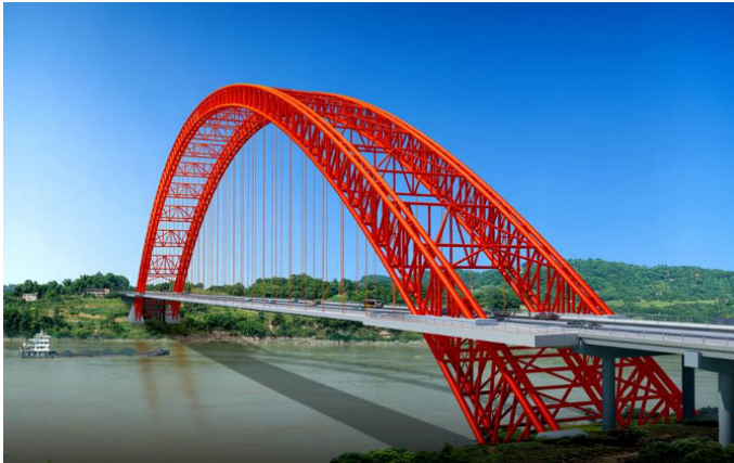
Fig. 1. Hejiang Yangtze River No. 1 Bridge, China.
