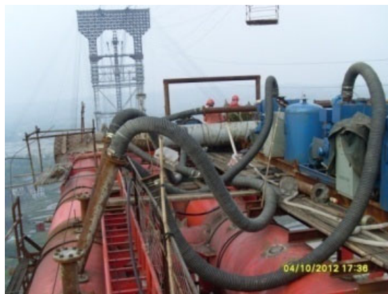
Fig. 11. The vacuum-pumping system on the arch crown of the real bridge.
