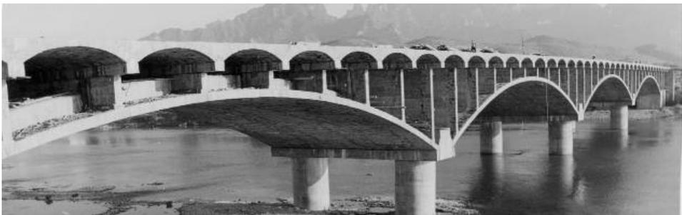
**Fig. 5.** Guanyin Bridge with coping of buttress, spandrel arch ring cantilevered  $2 \times 1$  m each, ( $2\Phi 3.5$  m hollow pier).
