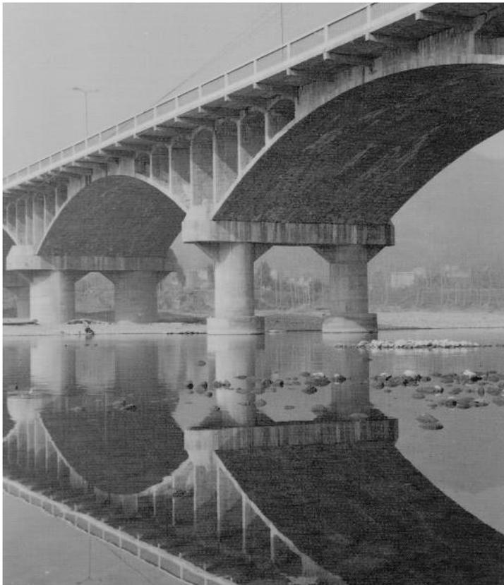
b) Guanyin Bridge with precast foot walk until cantilevered  $2\times 1$  m from the spandrel arch moreover, ( $2\Phi 4$  m/ $2\Phi 3.5$  m caisson digging pile)
