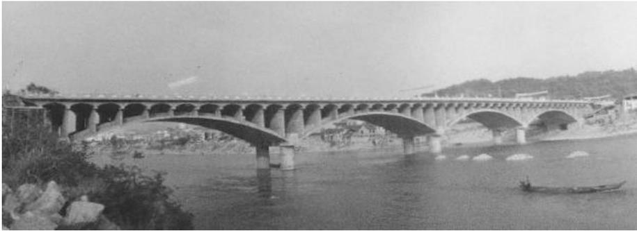
a) Lusiwan Bridge with cantilevered PRC beam for the deck structure, ( $2\Phi 3\text{m}-2\Phi 5\text{m}$  digging pile)
