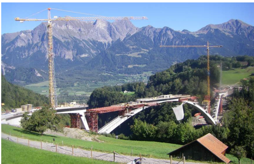
Fig. 9. Erection of the superstructure above the arch.
