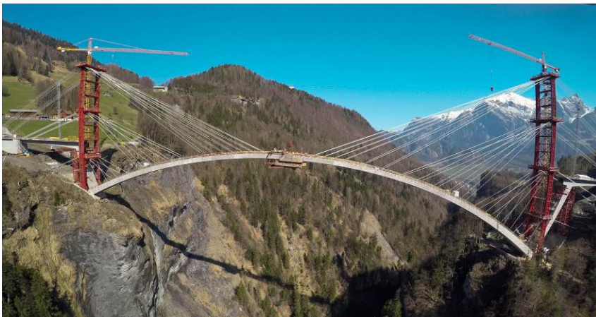
Fig. 8. Erection of the arch.
