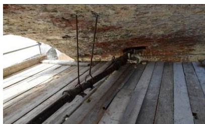
Fig. 2. Water pipe below the bridge – 2 nd half of 19 th century.
