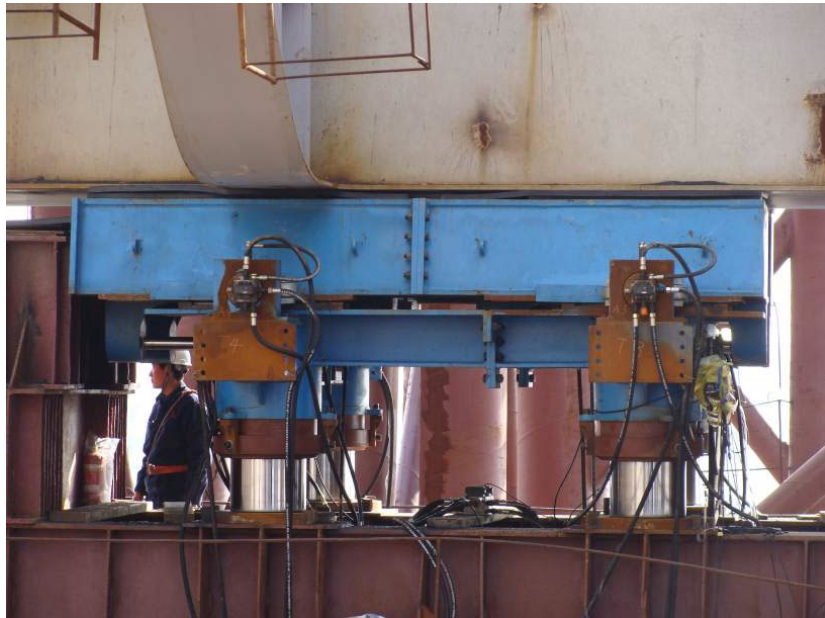
Fig. 6. the AWLS used in Jiubao Bridge construction.
