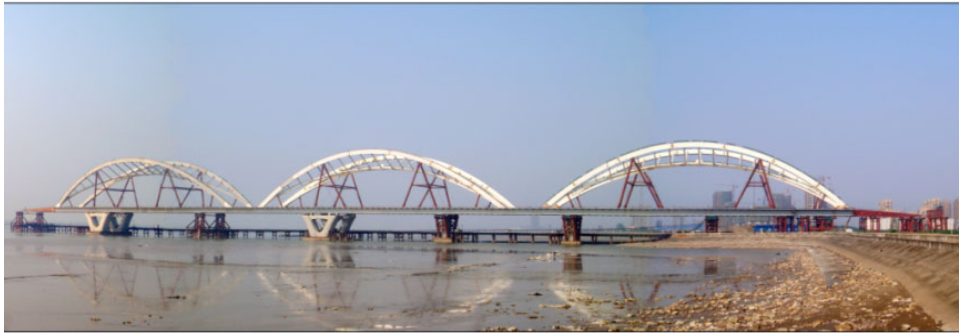
Fig. 10. Three spans of steel beam-arch structures under construction.
