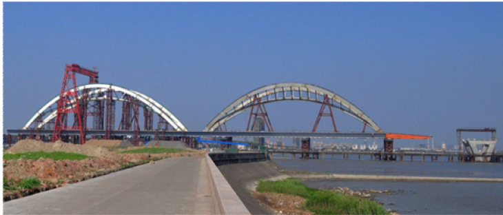
Fig. 3. Two spans of steel beam-arch structures.
