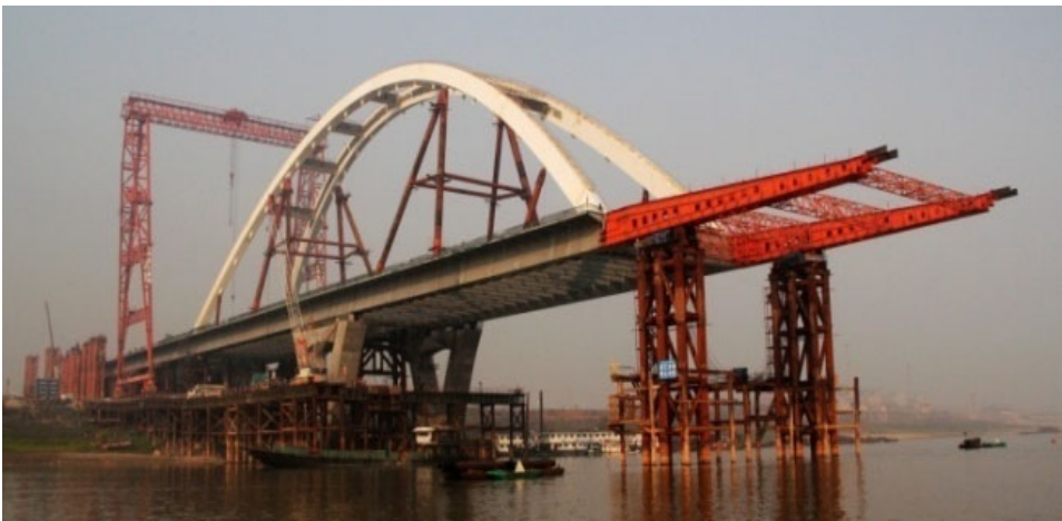
Fig. 13. The main span of Fuyuan Road Bridge under construction.
