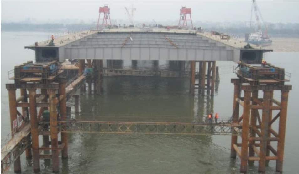
Fig. 12. Luozhou bridge under construction.
