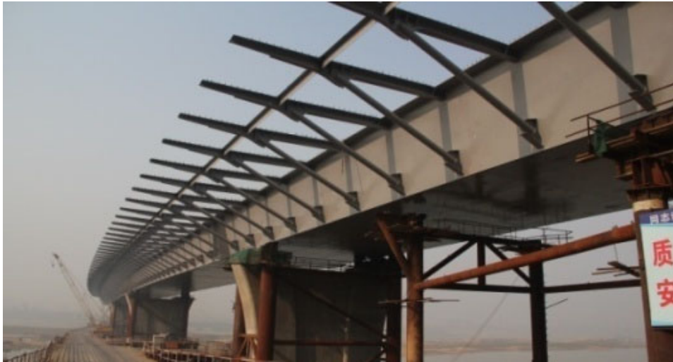
Fig. 14. The side span of Fuyuan Road Bridge under construction.
