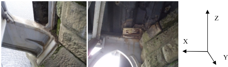
Fig. 6. Main Arch Rib end support & Top Chord end support (External Rib).
