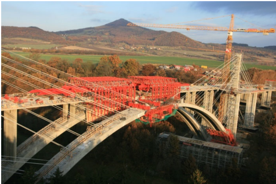
Fig. 3. Construction of the bridge.
