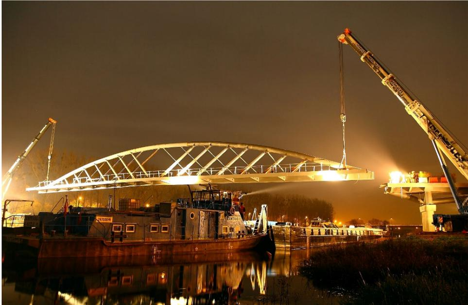
*Fig. 7. Erection of the main span (photo: Ryszard Bugaj).*
