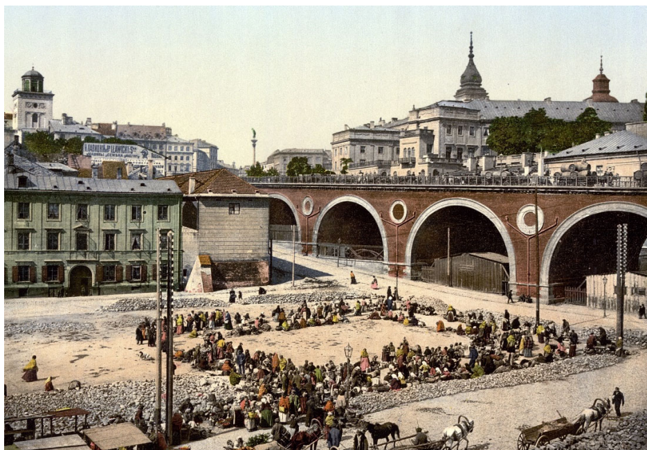
Fig. 3. View of the Pancer's Viaduct in Warsaw (photo: J. Biliszczuk's private collection).
