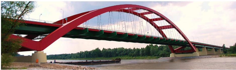
Fig. 1. General view of the Puławy Bridge (www.vistal.pl).
