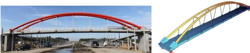
*Fig. 1. Arch footbridge mode shapes over the expressway S8 [photo MSC. Eng. Maciej Malinowski] altogether with visualisation of numeric model [6].*
