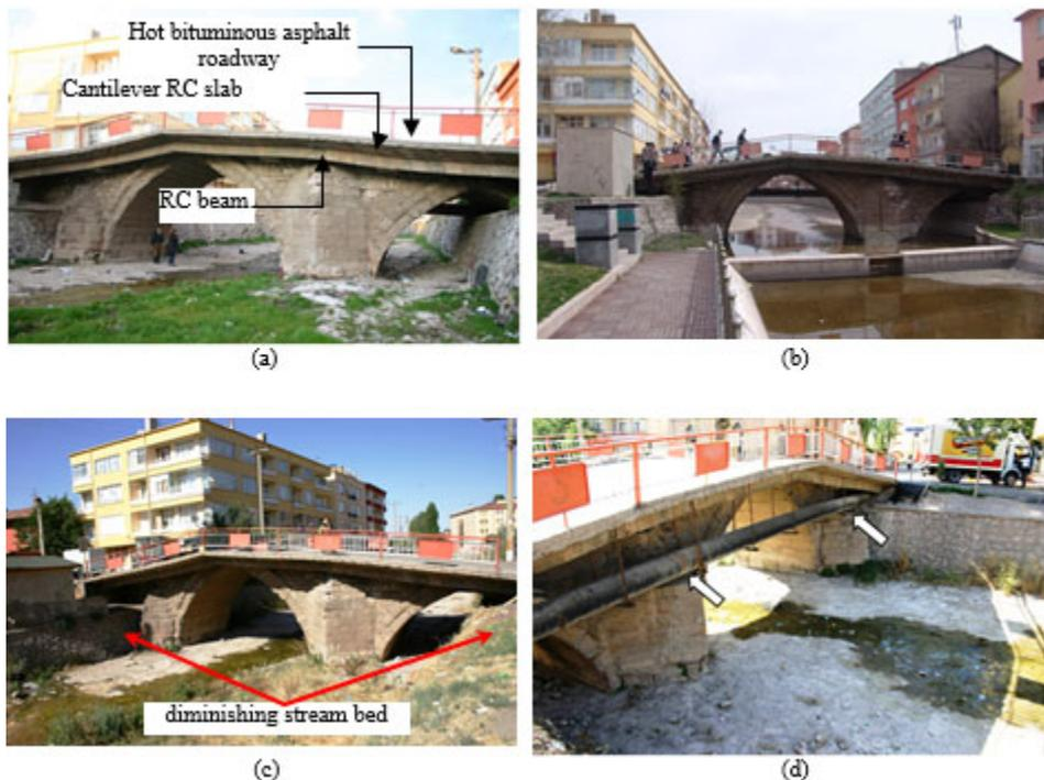
*Fig. 2. Former case, additions, and some damages of the bridge.*
