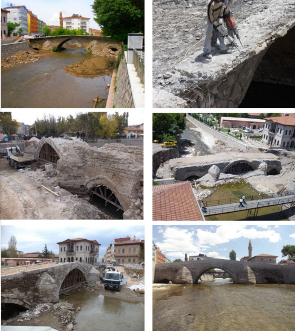
Fig. 5. Restoration stages of the bridge.
